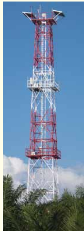
“Eddy Covariance Tower” to measure carbon flux in the ecosystem
